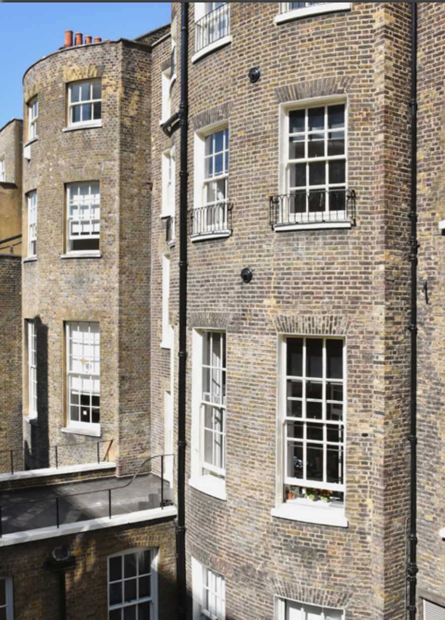
View from the AA Terrace, April 2018
