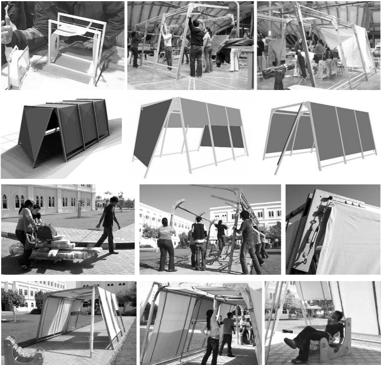
Fig. 3: Design, making and testing of the lightweight transitional structure.
