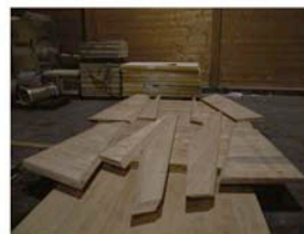
16. The panels were numbered and laid out. The quality of each cut was checked, and the panels themselves were checked against the original 3D model to ensure all pieces matched.
