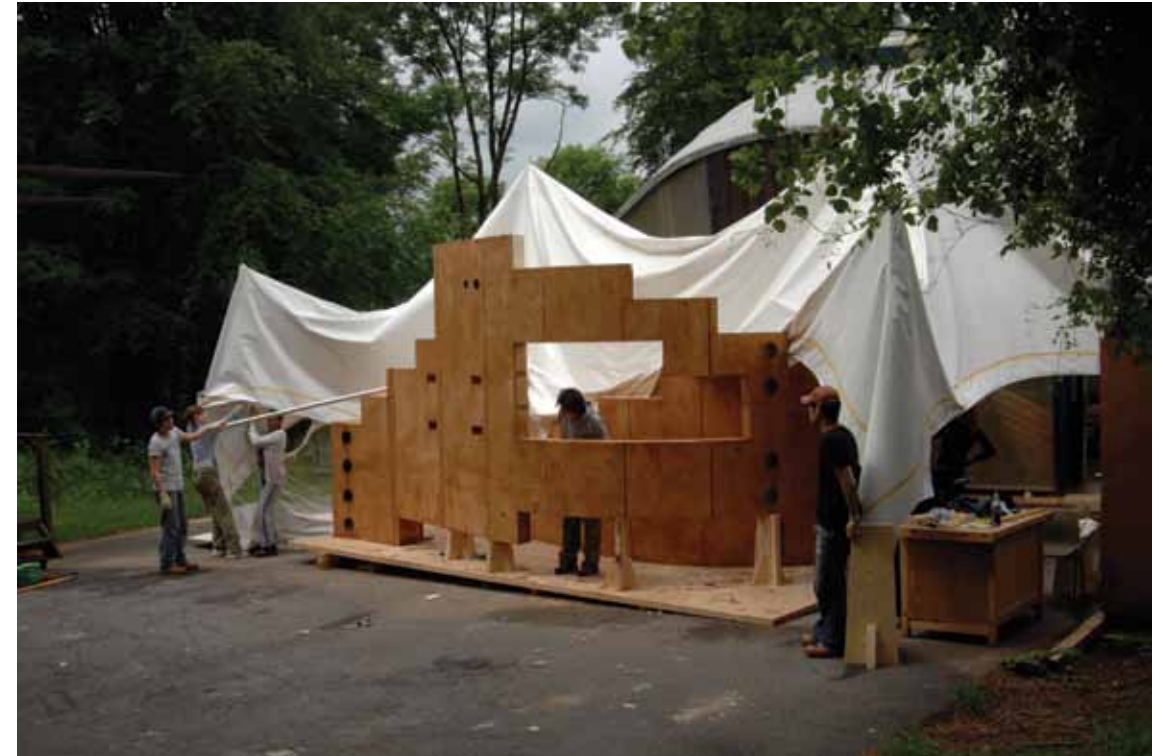
Stressed-skin box-beam component of 'Driftwood', the 2009 AA Summer Pavilion. Photos Valerie Bennett
